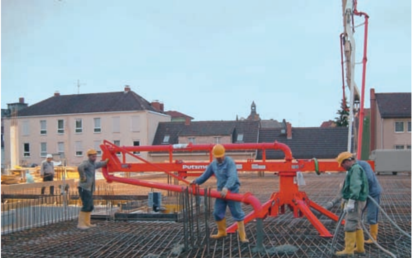
The RV 10 extends the horizontal reach of every truck-mounted concrete pump
